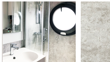
Badrum/ Bathroom: Formica Elemental Ash
